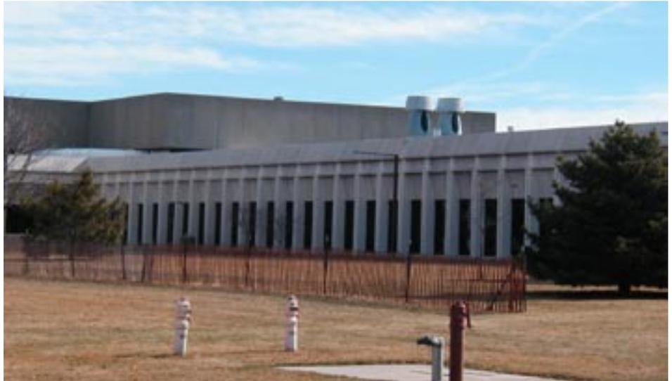
*Low profile mixed flow impeller exhaust systems on building roofs are aesthetically pleasing, and may help comply with applicable building codes as well as eliminate negative implications associated with tall exhaust stacks.*
