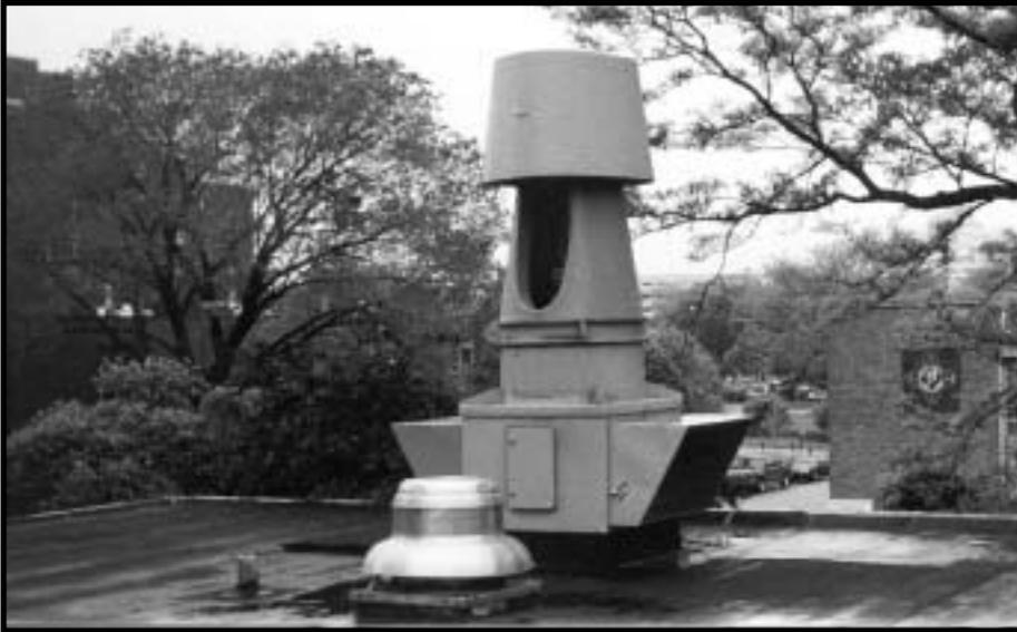
*Tri-Stack system is maintenance-free and provides an exhaust plume equivalent to an effective stack height of 35 feet.*
