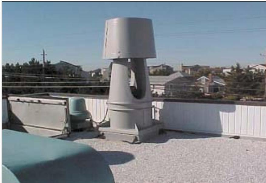
A mixed-flow impeller system mounted on the roof of a wastewater treatment facility treats odors through dilution.
