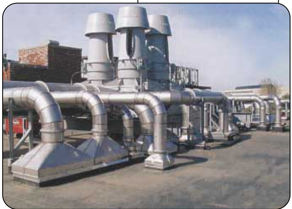
Elimination of exhaust re-entrainment possibilities, quiet operation, and prevention of toxic, noxious, or odoriferous workstation exhaust in the neighborhood were key requirements in the upgrading of the College of Veterinary Medicine's lab at Iowa State University. A roof-mounted, mixed-flow impeller exhaust system was selected to meet the lab's needs.
