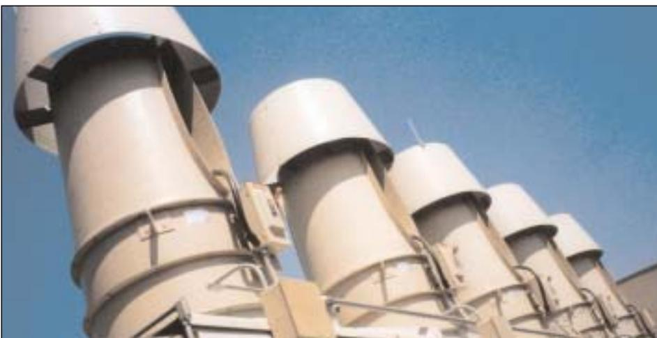
Fig. 3. TS series mixed-flow impeller fans connected to laboratory workstation fume hoods.
