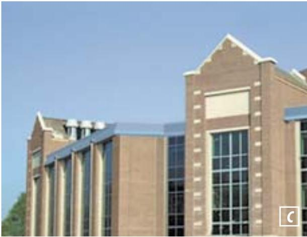
**On the cover . . .** At **Stanford University's Keck Science Building**, Palo Alto, California, eight Tri-Stack fans replaced 12 centrifugal fans for added performance and energy savings. The Tri-Stack fans are set in "quads," with each quad containing one operating fan and one standby; each fan provides approximately 25,000 CFM. New Strobic acoustical silencer nozzles are incorporated on four of the fans, with plans to retrofit the others as well.
