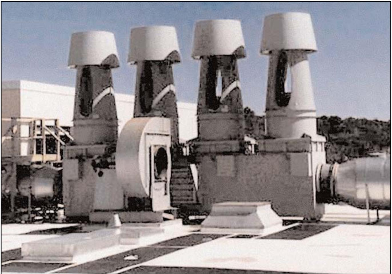
A ganged hood exhaust with an idle blower (foreground) that was removed after the photo was taken.
