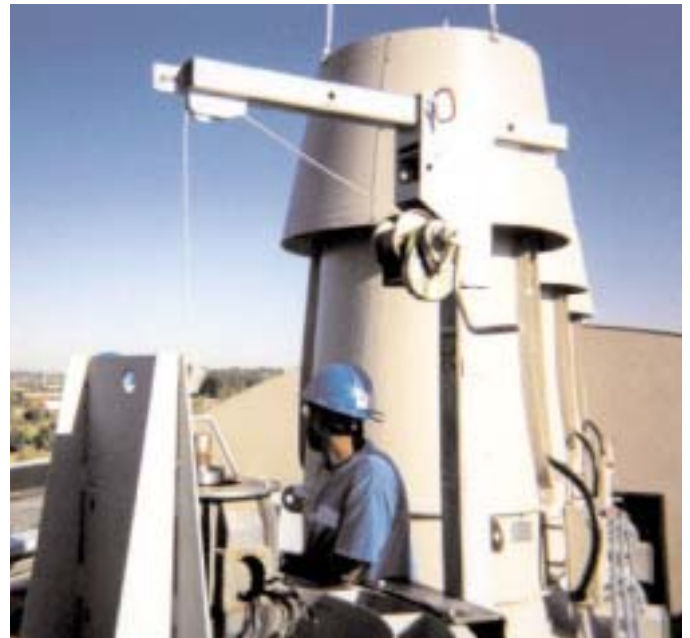
Align carefully over rotor. Replace shim and bolts. Rewire and test.
