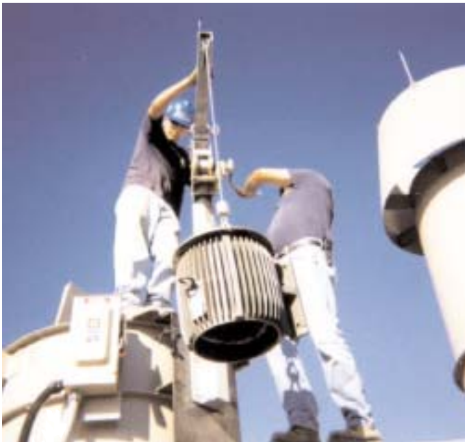
Lift new stator into place.
