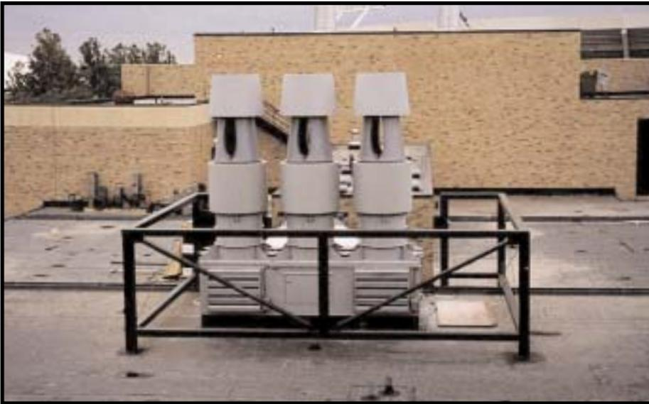
*Inline silencers were placed between the fan and exhaust stack to minimize airborne sound.*
