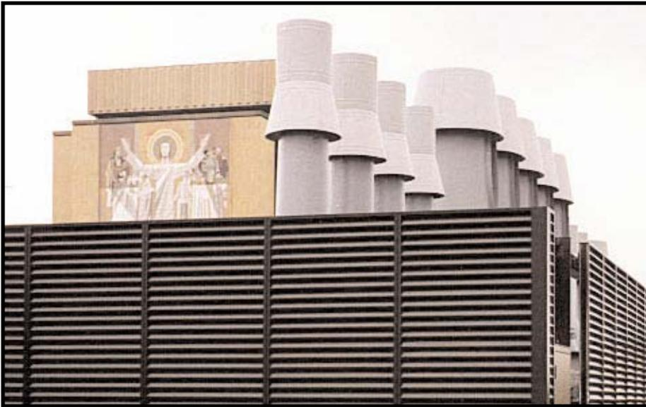
Acoustical architectural screen was placed around exhaust systems to minimize transmission sound.
