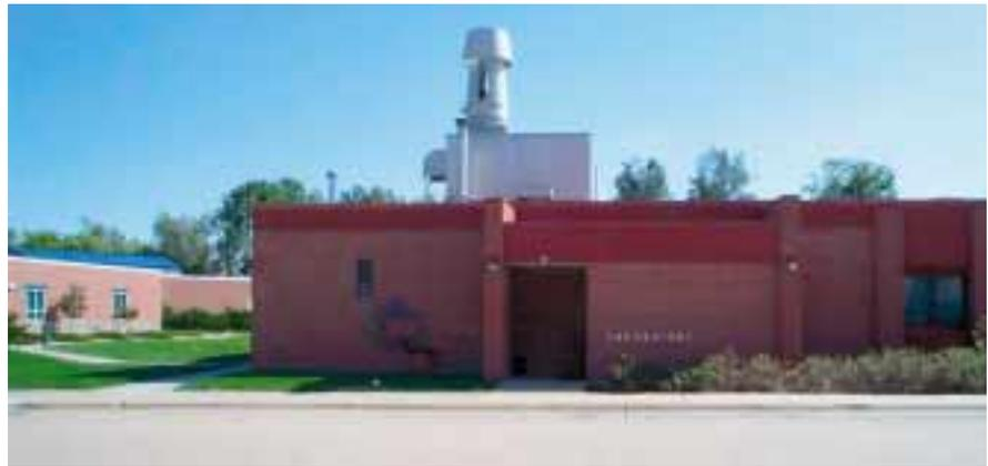
*MIXED FLOW IMPELLER FANS WITH HEAT RECOVERY MODULES at the Theresa Street Wastewater Facility prevent laboratory workstation fume hood exhaust from reentering the building, eliminate neighborhood odors, and significantly reduce costs for heating fuel.*
