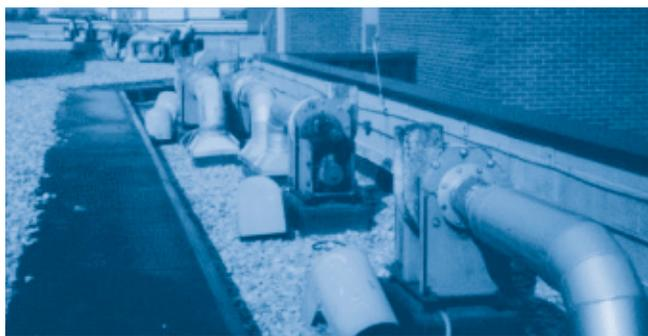
**The centrifugal fans on this roof (with their housings removed) require monthly drive belt inspection, according to ANSI Z9.5 Standards. Mandatory maintenance adds costs and downtime, while possibly exposing workers to dangerous fumes.**
