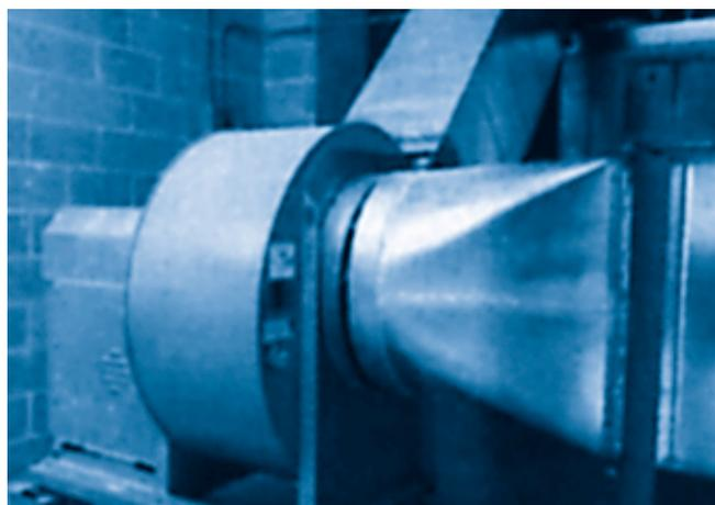
**Centrifugal fans such as this complex installation are highly susceptible to inlet and outlet system effects, with corresponding losses in performance efficiency.**
