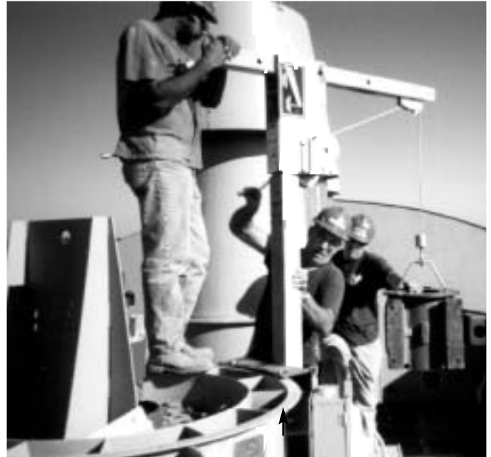
Attach jib to side of fan housing. Remove back endbell and stator.
