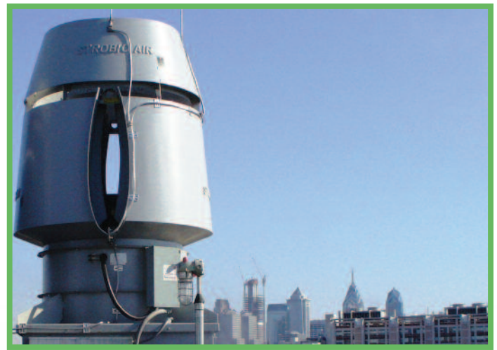
Patented Acoustical Silencer Nozzle and Acoustical Wind Band®
