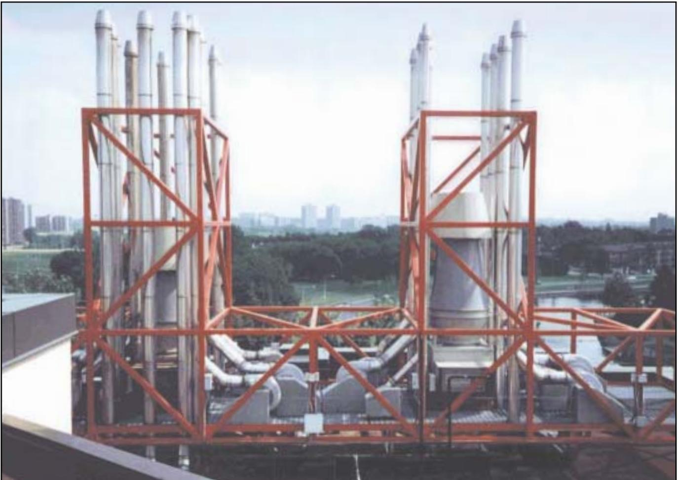
**Figure 1** The Strobic Air Tri-Stack system (surrounded here by individual centrifugal fan exhaust stacks from individual fumehoods) handles exhaust from 16 laboratory fumehoods through a common plenum on the roof.
